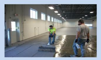
After the floor is shot blasted, the primer coat is applied. Then a 1/4"- high density epoxy floor mortar is installed.
