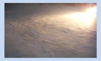
The Solution: Using a closed system shot blast machine, ESPOSITO LLC mechanically prepared the substrate by shot blasting the existing concrete to achieve the proper profile for maximum bond strength. ESPOSITO LLC installed a high density epoxy mortar floor system and abrasion resistant coating.
